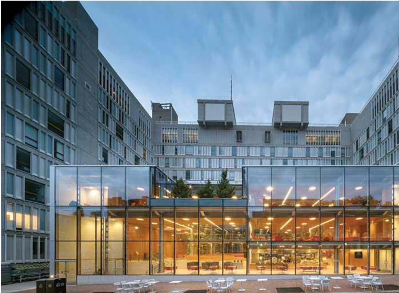
A glass-and-steel insertion fills in a courtyard of Sert's original administrative building for the school, adding a multilevel
