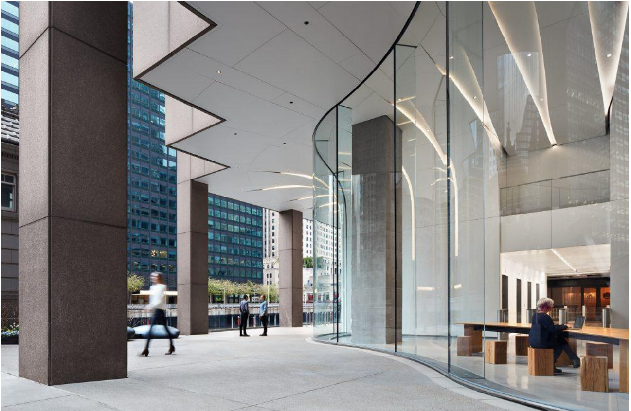
The structural glass curtain wall undulates between the preexisting granite columns. (Kendall McCaugherty/Hall + Merrick Photography)
